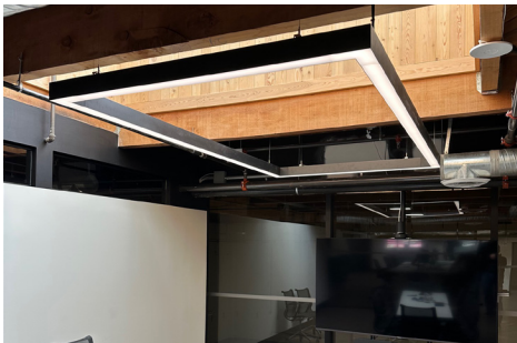
AL4-D-40W-3CCT-UD-BK 40W | 3CCT | 120-347V | Direct | 4608 lm AL8-D-80W-3CCT-UD-BK 80W | 3CCT | 120-347V | Direct | 9263 lm
